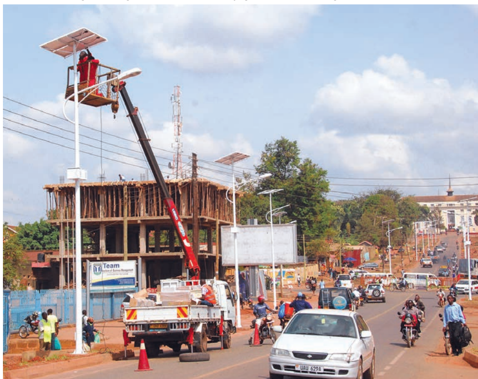
(below) Street lights being installed at Kabakanjagala Road in Rubaga Division
